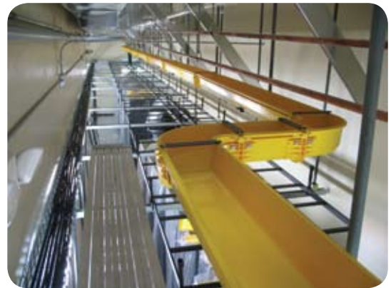
2G installed ADC's FiberGuide® Fiber Raceway System to route, manage and protect their fiber connections
